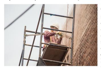
The work of tuckpointing is messy. The grinders that remove old mortar can be noisy and dirty. To minimize the amount of dust penetrating the building's interior, your windows and those of the neighbors should be covered, and protection added to landscaping if possible. Some things to look for:
